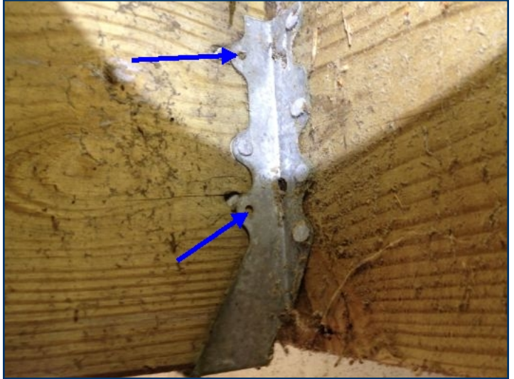
Missing nails in joist hangers
