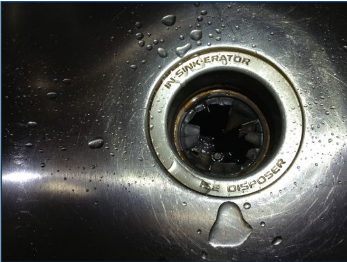
Splash guard broken.
