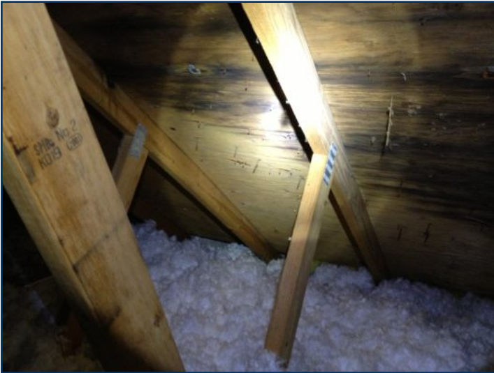
Notice the dark moisture staining on the sheathing
